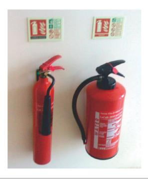
Figure 1.44 CO<sub>2</sub> and water extinguishers and information posters
